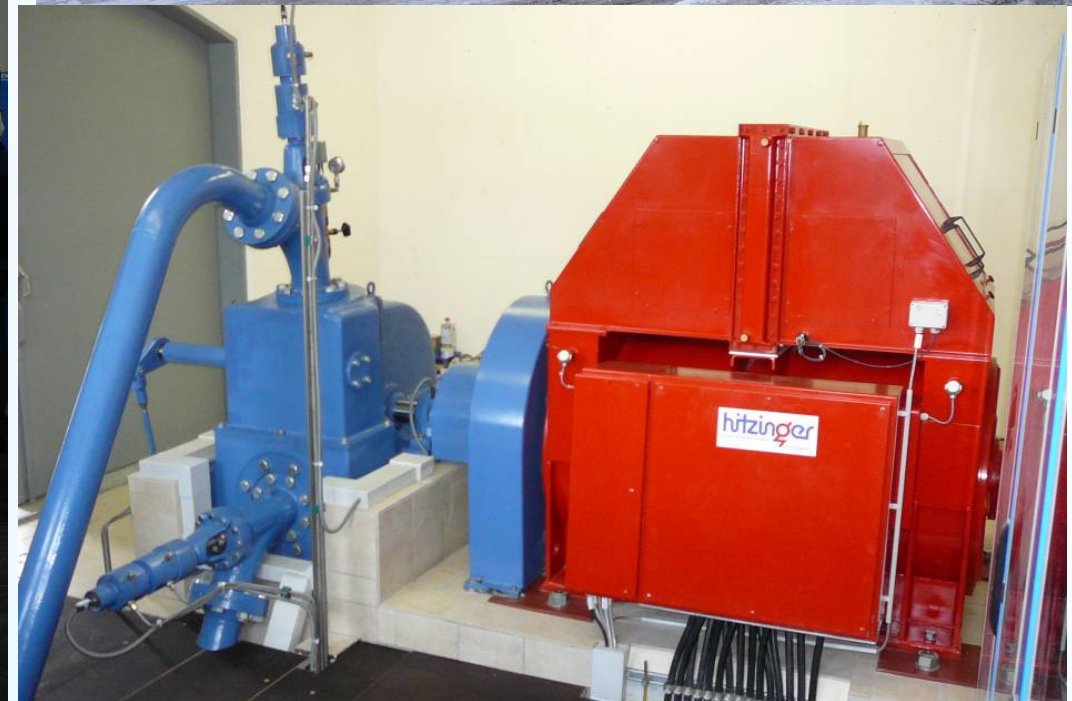
Synchronous alternator 830 kVA; weight 3,15 t, water cooled
